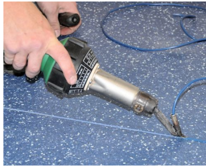
Figure : Heat Welding Vinyl Floor with Weld Rod
